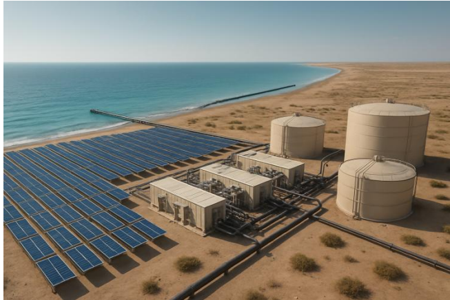
Fig. 8. Three-dimensional rendering of the solar-powered reverse osmosis facility, featuring photovoltaic arrays, RO modules, and storage tanks, is a 3D model of the Mocha desalination plant.
