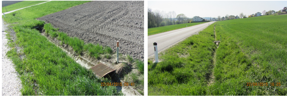
Figure 3: Roadside ditch with multiple storm drains at varying distances. The left picture was taken upstream of the right.
