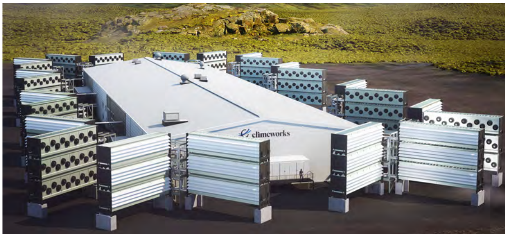
Figure 16.5: Climeworks, a Swiss company specializing in solid-sorbent direct air capture (DAC), has developed and operated a sequence of progressively larger plants in Europe and Iceland. In 2021 the company commissioned Orca in Iceland, the first industrial-scale DAC plant, with a nominal capacity of 4,000 \text{ t}_{\text{CO}_2} \text{ yr}^{-1} , powered by geothermal heat and electricity. This was followed in 2023–2024 by Mammoth , also in Iceland, designed as a modular array of twelve containerized DAC units with a projected capacity of 36,000 \text{ t}_{\text{CO}_2} \text{ yr}^{-1} once fully operational ( Climeworks AG, 2024 ). The company has announced plans for future hundred-thousand-tonne-scale facilities later in the 2020s, but as of 2025 its operating plants collectively capture well under 50,000 \text{ t}_{\text{CO}_2} \text{ yr}^{-1} – orders of magnitude below what would be required for any meaningful contribution to global carbon-removal targets. Image source: Climeworks, 2022.
