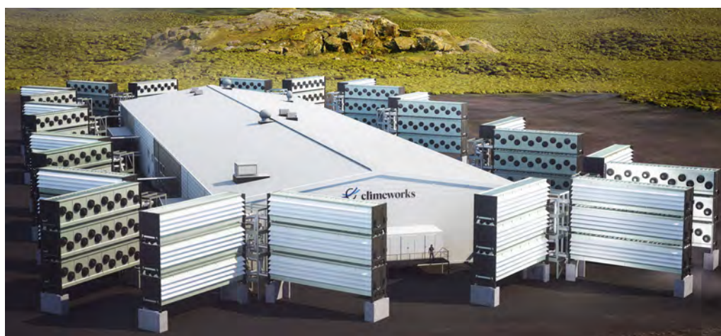
Figure 14.5: Climeworks, a Swiss company specializing in solid-sorbent direct air capture (DAC), has developed and operated a sequence of progressively larger plants in Europe and Iceland. In 2021 the company commissioned Orca in Iceland, the first industrial-scale DAC plant, with a nominal capacity of 4,000 \text{ t}_{\text{CO}_2} \text{ yr}^{-1} , powered by geothermal heat and electricity. This was followed in 2023–2024 by Mammoth , also in Iceland, designed as a modular array of twelve containerized DAC units with a projected capacity of 36,000 \text{ t}_{\text{CO}_2} \text{ yr}^{-1} once fully operational ( Climeworks AG, 2024 ). The company has announced plans for future hundred-thousand-tonne-scale facilities later in the 2020s, but as of 2025 its operating plants collectively capture well under 50,000 \text{ t}_{\text{CO}_2} \text{ yr}^{-1} – orders of magnitude below what would be required for any meaningful contribution to global carbon-removal targets. Image source: Climeworks, 2022.
