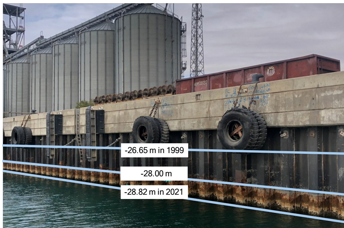
Figure 2: Photograph showing the changes in water levels at Aktau Port between 1999 and 2021 and the use of temporary fenders
