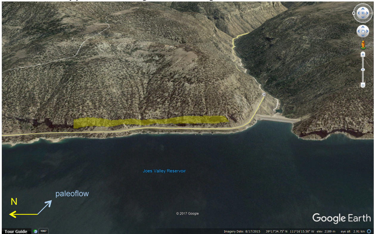
B. Joe's Valley panel location along the road bordering the reservoir.
