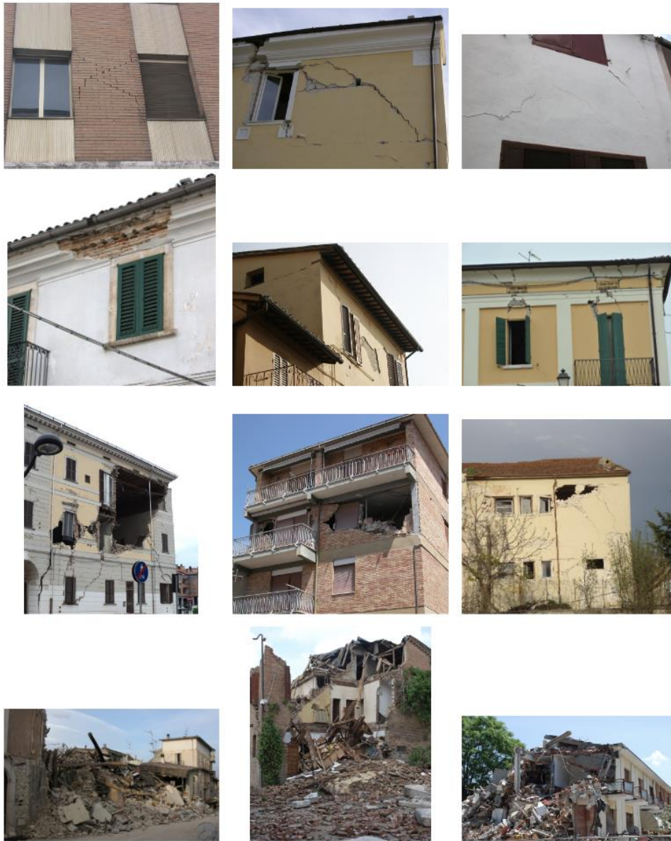
Figure 3. Sample images from the DFM test set illustrating the range of damage manifestations addressed by the MSM model. Rows correspond to increasing EMS-98 severity, from grade 1/2 (top row) to grade 5 (bottom row); columns illustrate the heterogeneity of acquisition geometries characteristic of opportunistic ground-survey photography. Images obtained from the INGV DFM.
