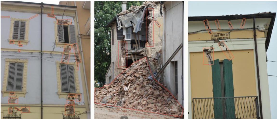
Figure 4. Examples of the mixed-geometry annotation protocol. Oriented bounding boxes are used for linear damage features (grades S1–S3), while polygonal masks are used for spatially irregular damage (grades S4–S5).
