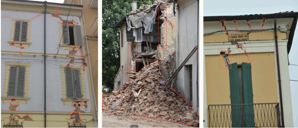
Figure 4: Mixed-geometry annotation protocol in CVAT.ai: oriented bounding boxes for the linear/sub-linear features of grades S1–S3, polygonal masks for the irregular extents of S4–S5, with all S1–S3 boxes converted to masks prior to training.
