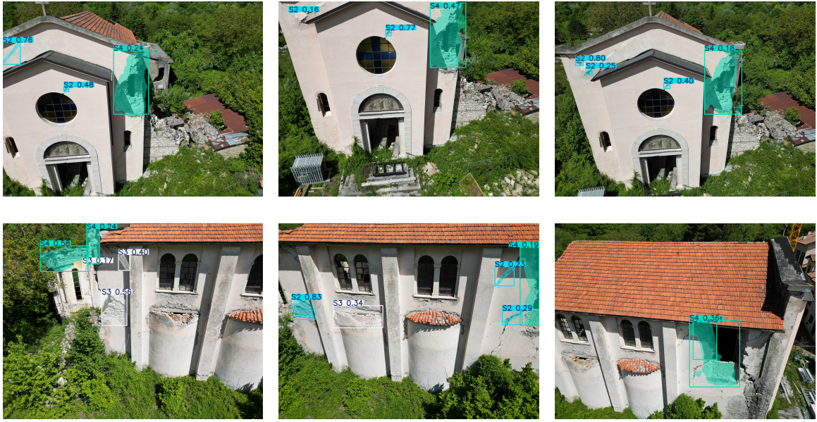
Figure 12: Multi-view attribution of the church (CODICE 337040_3349): six of the 35 UAV photographs used to classify the building, showing converging lines of sight on different façades. Per-image grades vary across S2–S4; the worst-observed aggregation rule resolves them into a single building-level \max\_grade = S4 .
