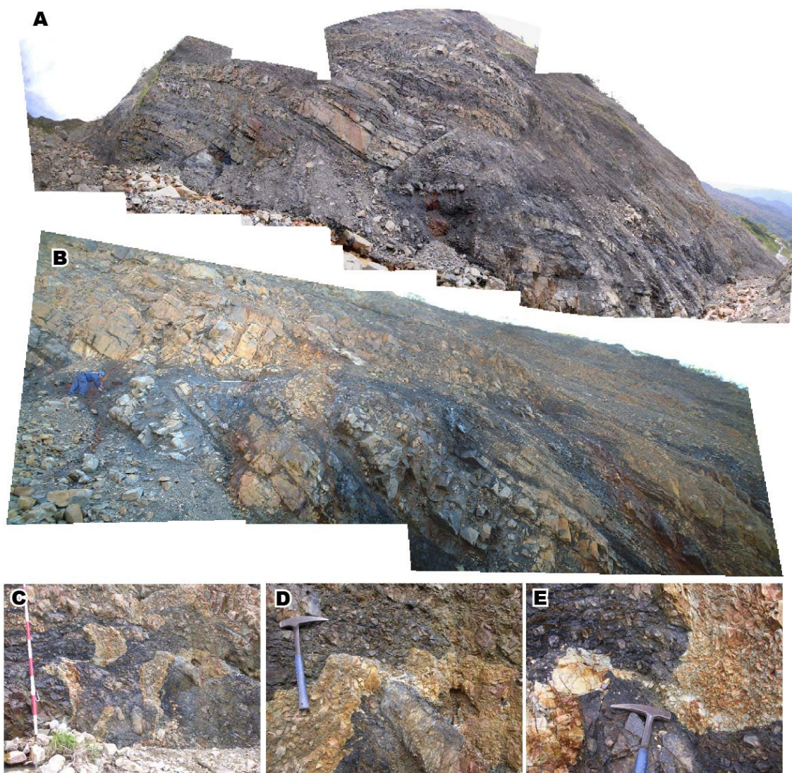
Figure 2. Geological and structural characteristics of the Jin'nosuke-dani landslide. (A) Large-scale view of the landslide mass. (B) Shale and sandstone beds exposed along the Betto-dani Valley. (C–E) Close-up views of sheared shale and clay-rich slip zones. The orientations of the principal shear structures are described in the text.
