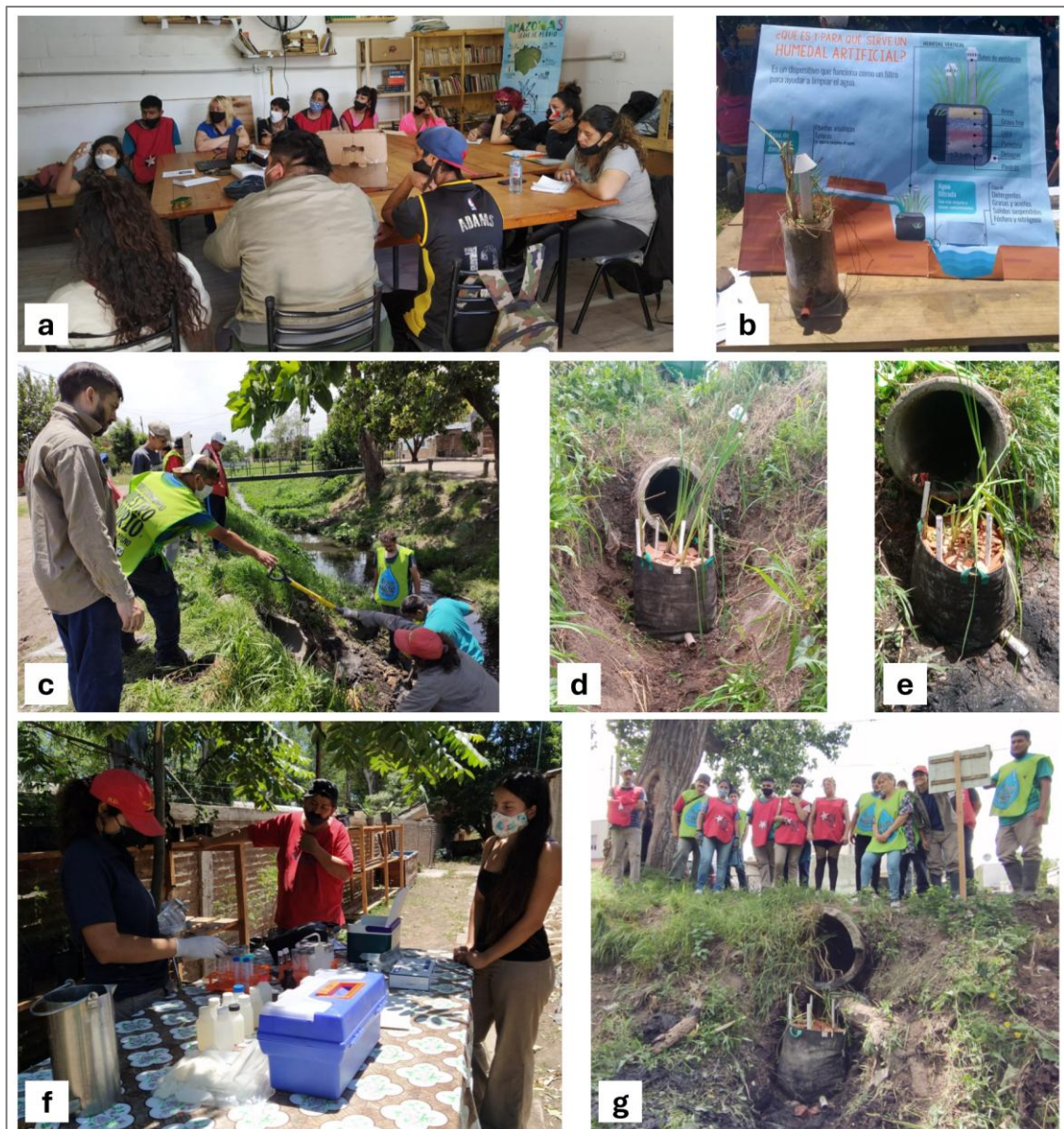
Figure 3. Co-production process. (a) Results discussion and planning workshop (November 8, 2021). (b) Infographics and model used in community outreach activities. (c) Site preparation and biofilter installation at stormwater drain outlets. (d–e) Installed biofilters in the field. (f) Mobile laboratory set up at the social organization's premises for nitrate and SRP determination. (g) PHC team that participated in installation events and sustained biofilter maintenance
