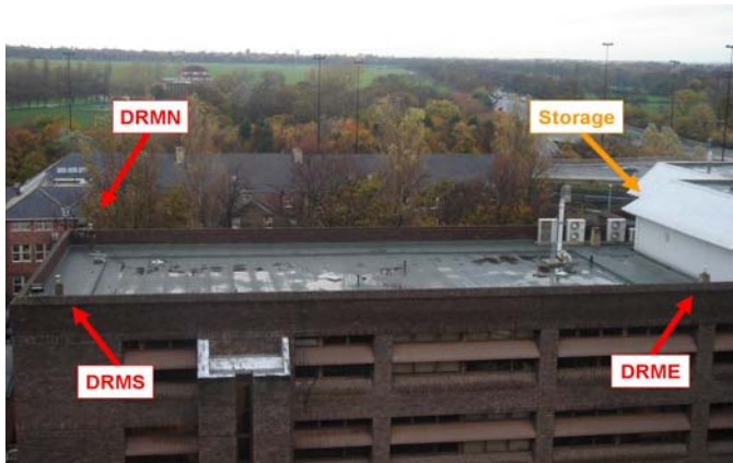
Figure 2. Relative location of the three Drummond building stations.
