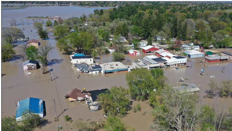
Figure 8: The aftermath of dam breaks in Michigan on May 19, 2020
