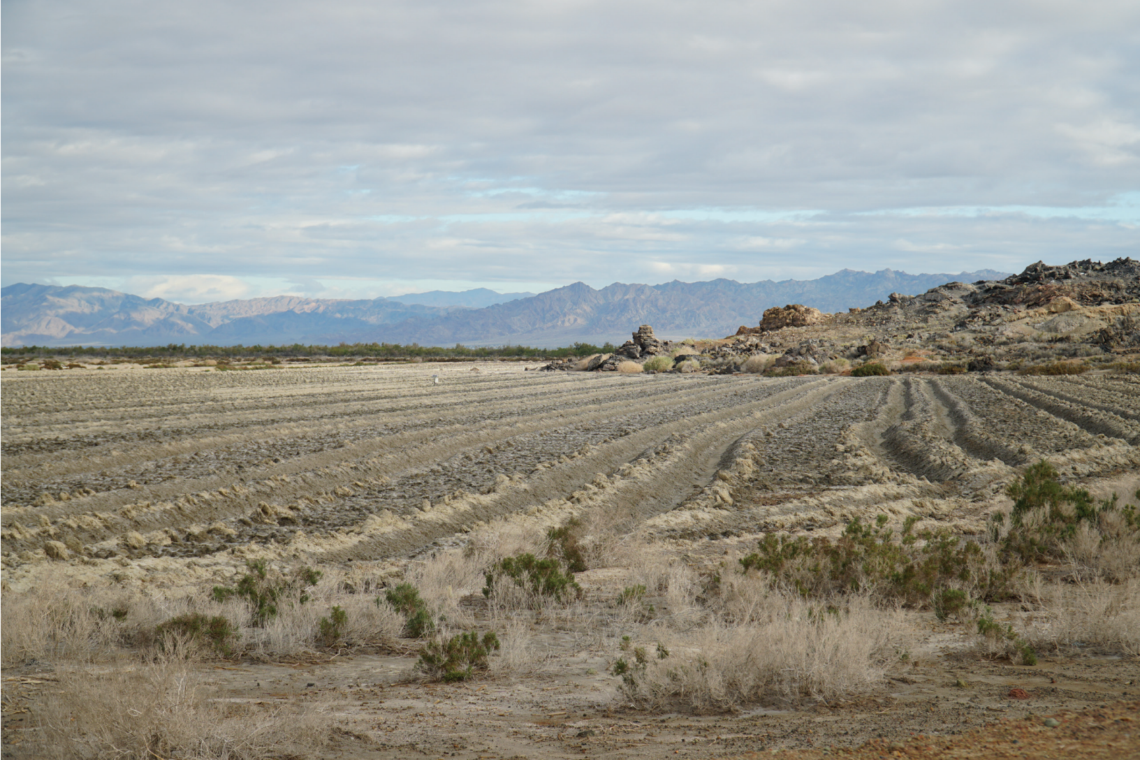
DUST BERMS constructed to reduce windblown dust along the exposed southern shore of the Salton Sea. Jonathan Nye
