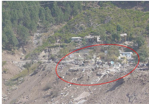
Slope failure caused damage to many buildings in Balakot
