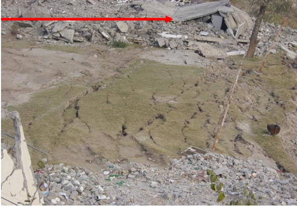
Destroyed Nisar Camp near Muzaffarabad close to rupturing zone
