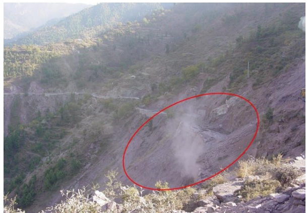
Fracturing and shaking caused major slides along the Kaghan road
