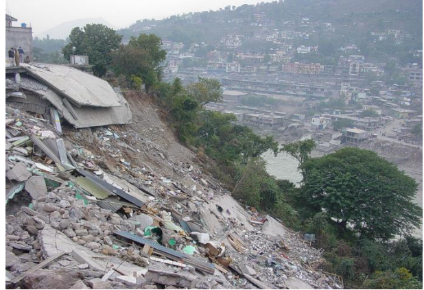
Slope/ soil failure in Muzaffarabad along with the River Neelum
