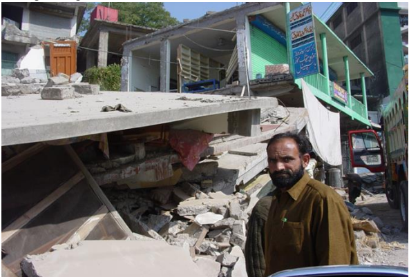
Collapsed improper concrete buildings in the foreground and light wooden structures in the background
