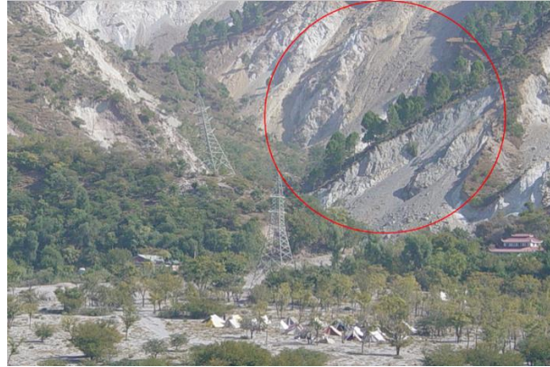
Rock sliding along a fault zone in Balakot area
