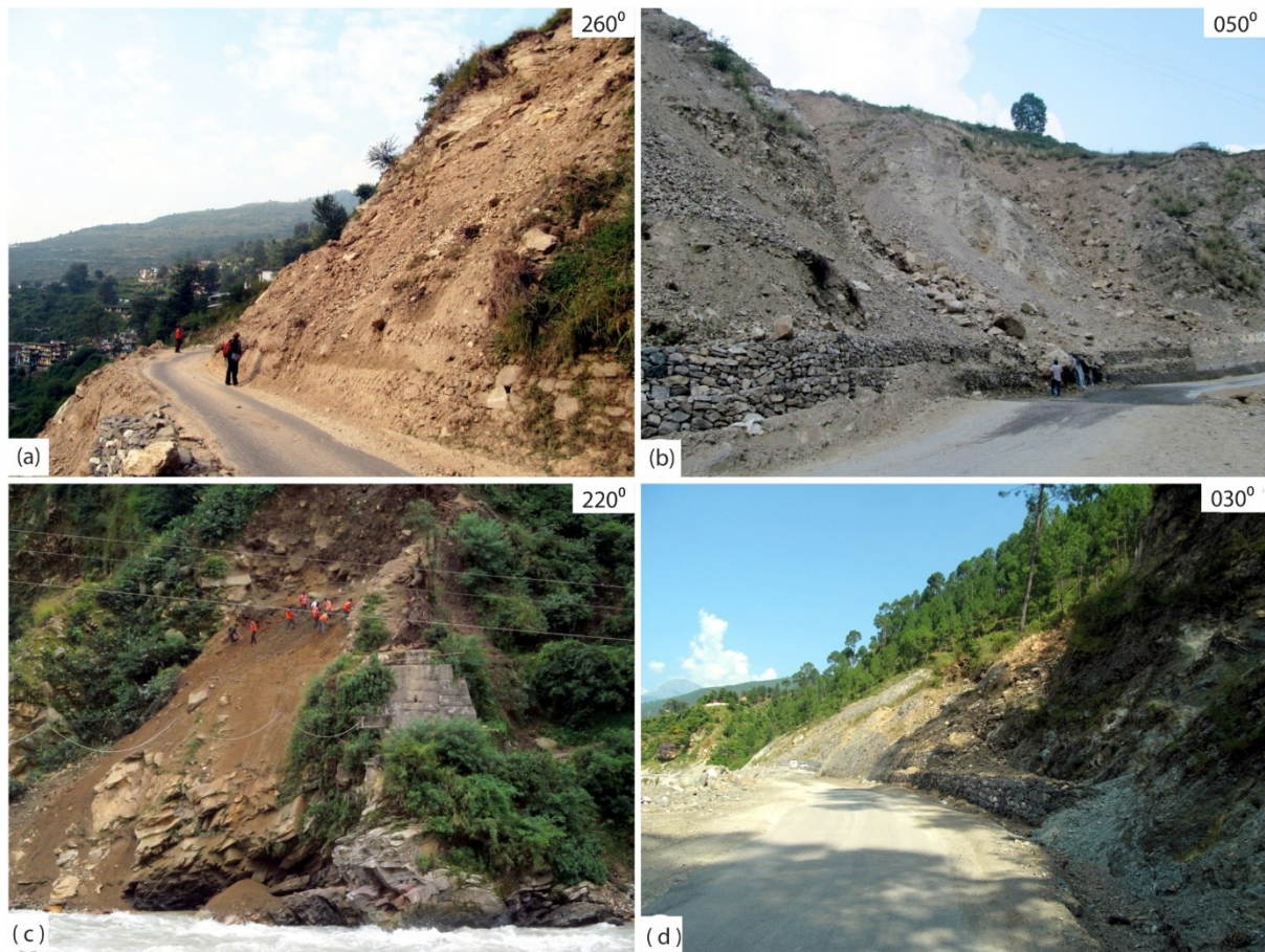
Repository Fig. 6: Landslides producing debris flow from the Garhwal Lesser Himalaya. Debris material contains soil and rock fragments (up to boulder size). (a) in MCT zone schists and quartzites at 30.8136^{\circ} N, 78.6205^{\circ} E, Location 1 also known as Lata ghatori slide in Fig. 5 . (b) At Munsuari Thust footwall at 30.7725^{\circ} N, 78.5997^{\circ} E, Location 6 in Fig. 5 . (c) Within Berinag Formation quartzites at 30.76^{\circ} N, 78.5811^{\circ} E, at location 8 in Fig. 5 . (d) within quartzites of Berinag Formation at 30.7544^{\circ} N, 78.5593^{\circ} E, near location 4 in Fig. 5 , also known as Ganeshpur slide.
