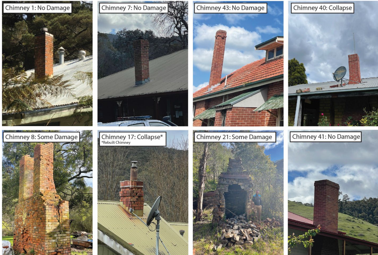
Figure 5: Photos of chimneys with various damage states post the Woods Point earthquake.
