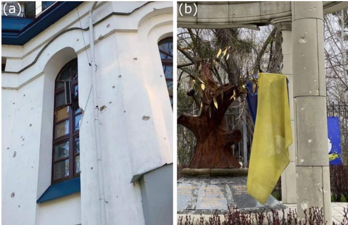
Figure 1: (a) Shrapnel damage to the facade of the St Nicholas Church caused by Russian shelling in the town of Irpin, a suburb to the NW of Kyiv in Northern Ukraine (2). (b) Impact damage to columns of the Alley of ATO Heroes memorial, also in Irpin. It is reported to have been fired upon intentionally by Russian forces in February 2022 (1, 2).
