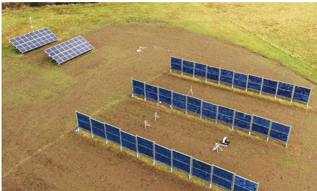
Figure 3. Aerial picture of the first agrivoltaic system in Sweden comprising of three vertical bifacial PV rows. Photo credit: IVAR Studios AB.
