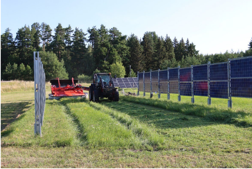
Figure 6: Vertically mounted APV system during the first cut in 2021 and reference CGMPV system in the background.
