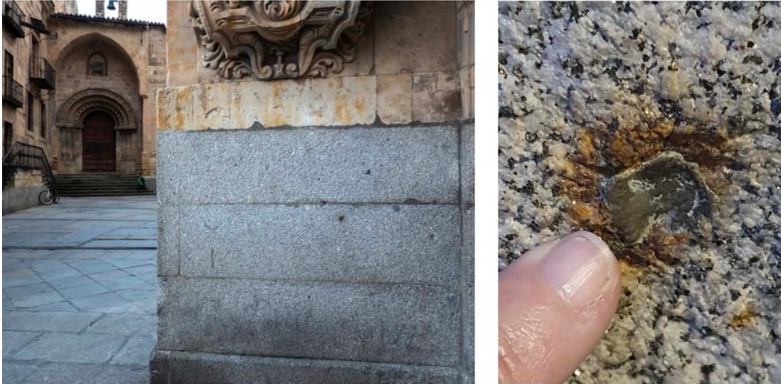
Figure 5. Dark spots in granite, due to small iron-rich enclaves, which were interpreted as marks left by the shooting. Even if the explanation is not true, history allows us to recall a very tragic event at the beginning of the war. Picture courtesy of Vicente Sierra Puparelli. Right: Detail of one of the dark spots. Picture by the author.
