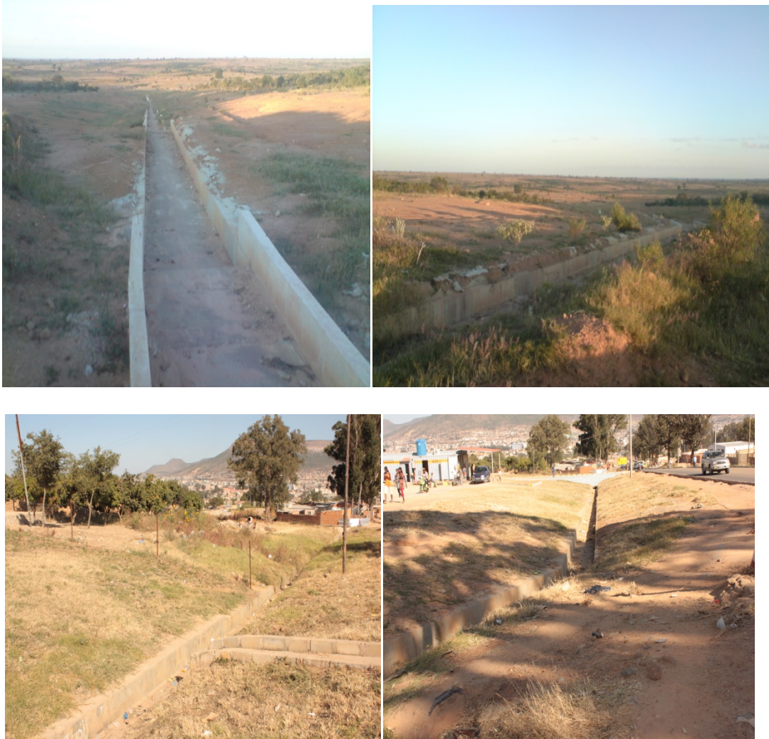
Figure 9: Image of four ditches built in Lubango to channel excess water from heavy rains. An example of possible low-impact best practices to be implemented in Las Loras Geopark as preventive measures. Source: Armanda Cruz, 2011.
