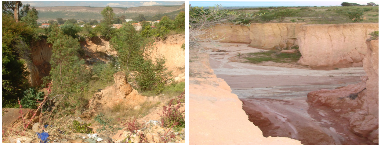
Figure 8: Consequences of floods that affected roads and paths and caused landslides in the surroundings of Lubango. Source: Armanda Cruz, 2011.
