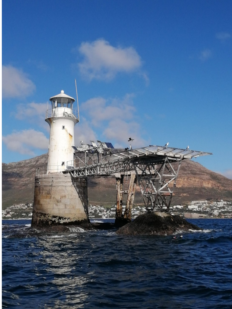
Figure 2.: Roman Rock lighthouse – December 2022. The cast-iron lighthouse was built in 1861 on top of a granite tor that protrudes above the sea surface at low tide. Note the north-facing solar panels that power the lighthouse. Simon’s Town appears in the background at the base of the 678m high Swartberg mountain. Image credit: Andrew Morson.
