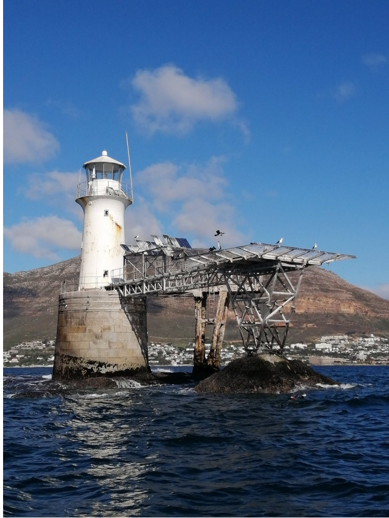
Figure 2. Roman Rock lighthouse – December 2022. The cast-iron lighthouse was built in 1861 on top of a granite tor that protrudes above the sea surface at low tide. Note the north-facing solar panels that power the lighthouse. Simon's Town appears in the background at the base of the 678m high Swartberg mountain. Image credit: Andrew Morson.
