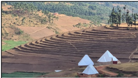
A: Radial bench terraces, constructed with earth movement
