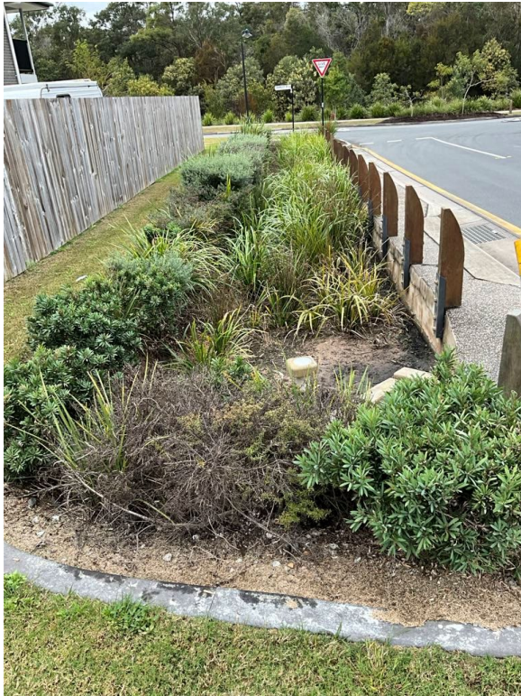
Figure 6 Street scape bioretention
