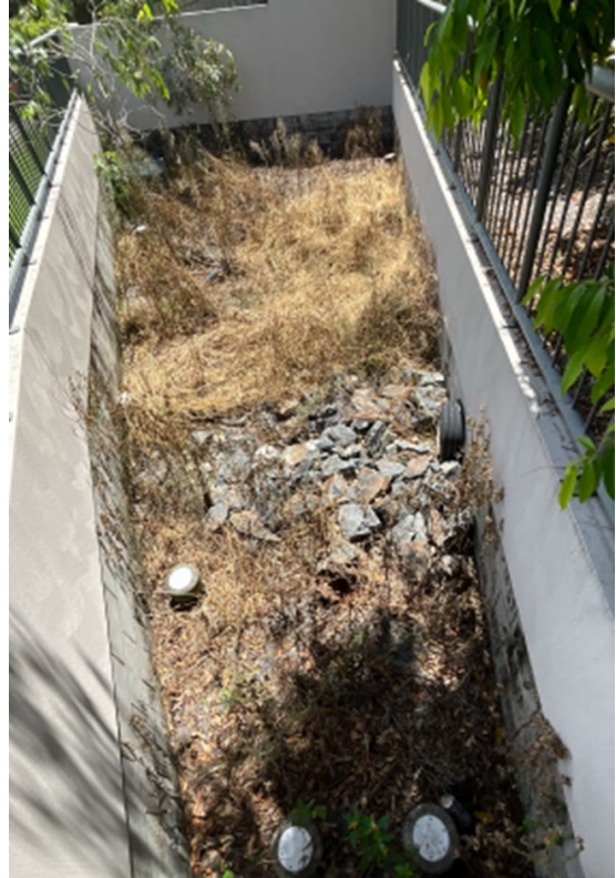
Figure 5 Examples of failed and neglected / mismanaged biobasins without amenity provision
