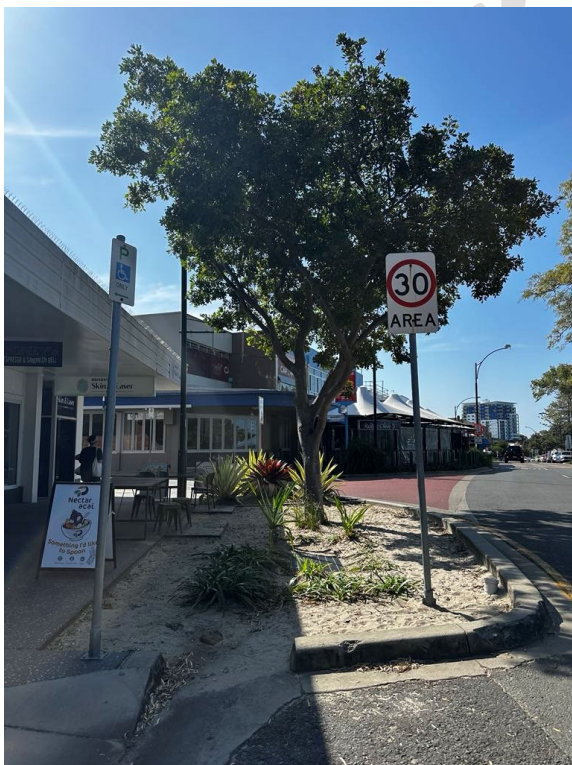
Figure 8 Civic space bioretention system
